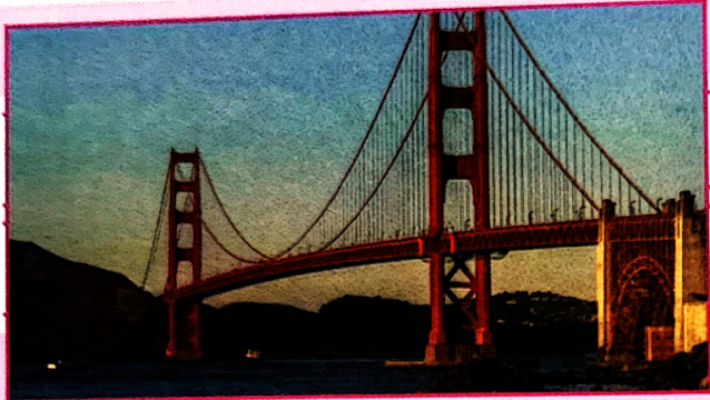
Golden Gate Bridge
